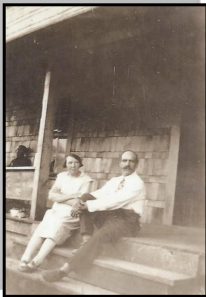
Maggie & Ransom Higley at the Quinault Hotel on the South Shore. Circa 1906. Note the 2"-5" shingle pattern on the wall, common to that era. The Museum also has that pattern.
